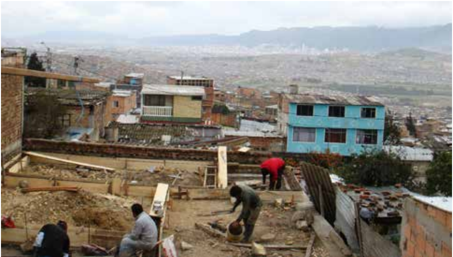
Building a new home in Bogotá
